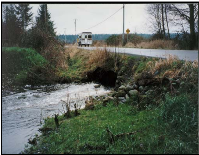
Little River crossing after construction
