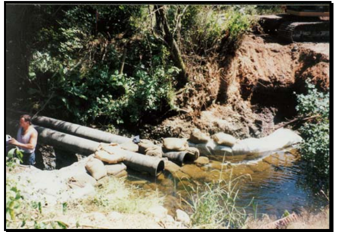
Little River crossing during construction
