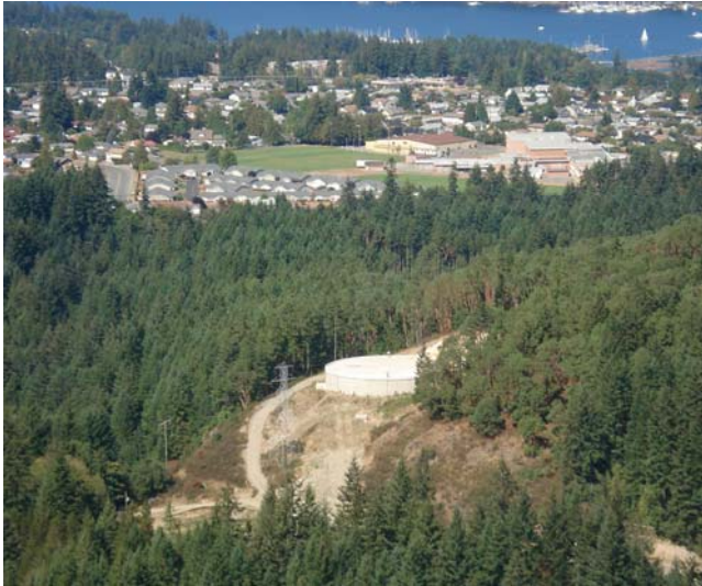
View of the new Arbutus Reservoir with Town of Ladysmith and harbour in background
