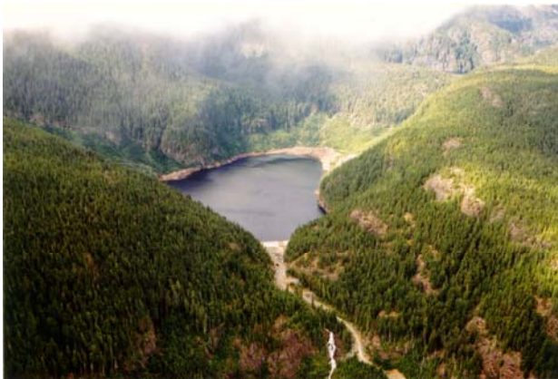
Aerial View of Arrowsmith Lake, dam, and outlet channel Elevation 800 m
