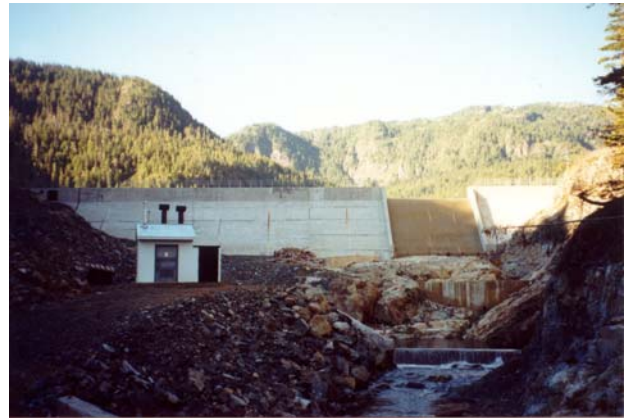
Completed dam, showing spillway, generator building and outlet/spillway channel.
