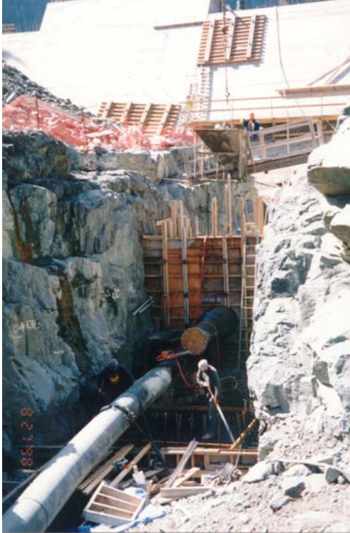
Outlet piping in rock trench, with dam construction in background.
