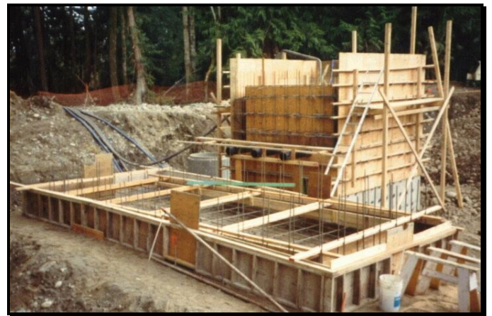
Formwork for the valve chamber and wet well
