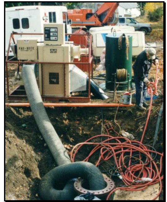
Dehumidification equipment used to cure the applied coating material
