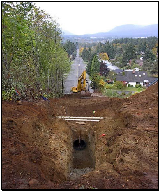
Water Main Installation
