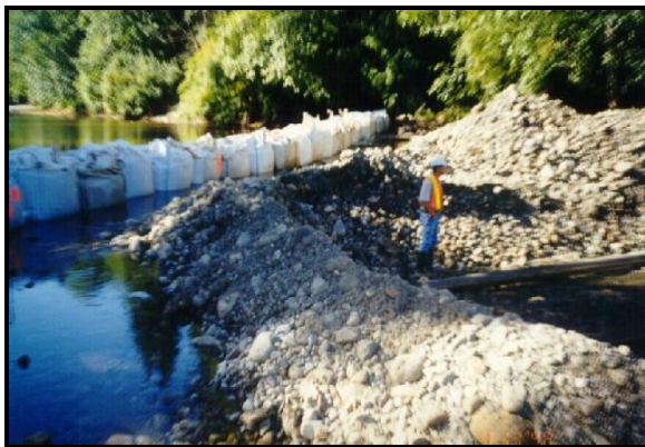
Infiltration gallery excavation
