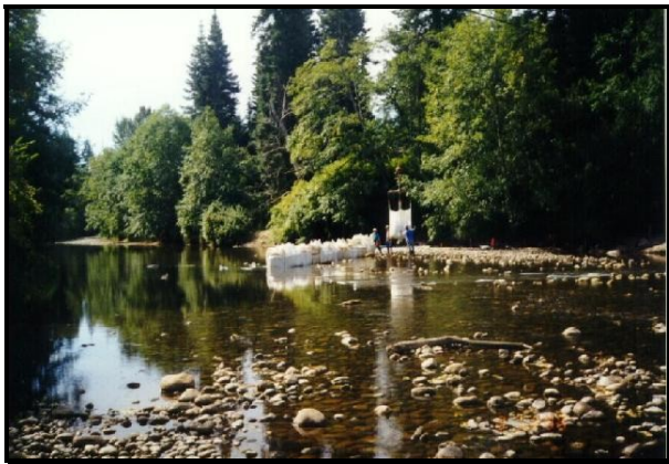
Installing the river diversion for the new infiltration gallery
