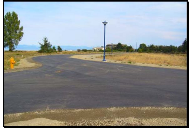
Completed 13 Lot strata site
