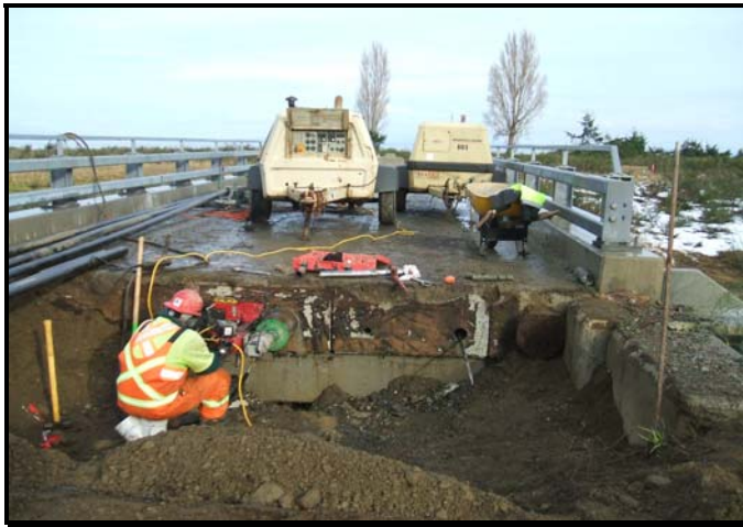
Utility coring through the bridge crossing at Little River.
