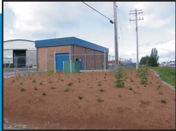
Completed Labieux Road Booster Station
