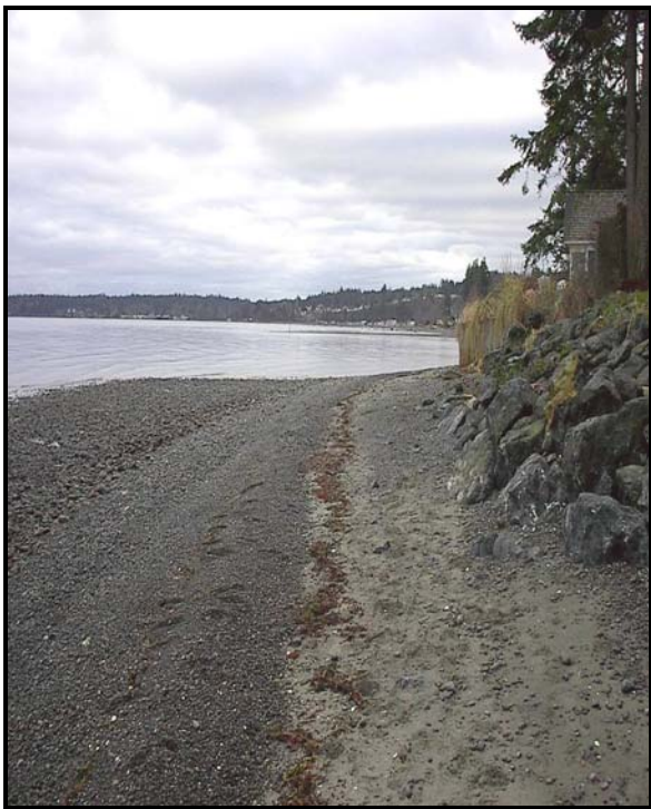
Foreshore condition after force main installation
