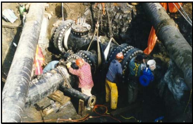
The new 610 mm dia. supply main following tie-in to the existing 900mm dia. watermain underneath the two fish hatchery supply mains.
