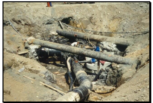
The new 610 mm dia. supply main following tie-in to the existing 900mm dia. watermain underneath the two fish hatchery supply mains.
