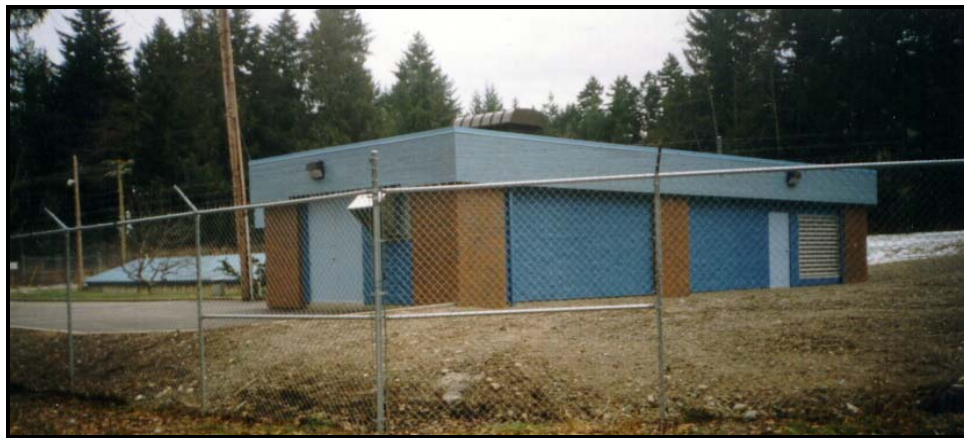
View of the Springwood compound, showing the expanded pump station with the low level reservoirs in the background
