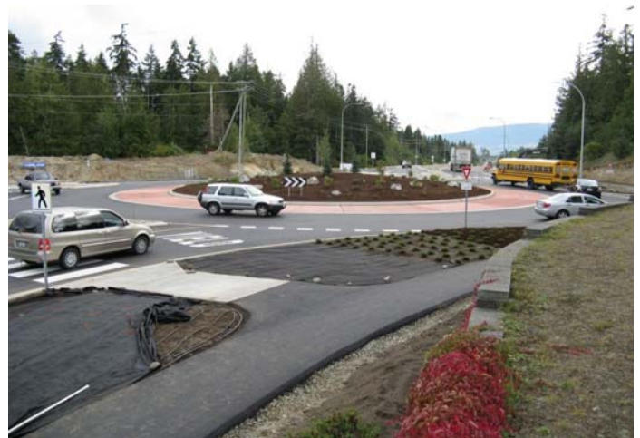
Roundabout functioning as designed. Note the low profile landscaping (in progress) to provide an attractive entrance and good visibility.
