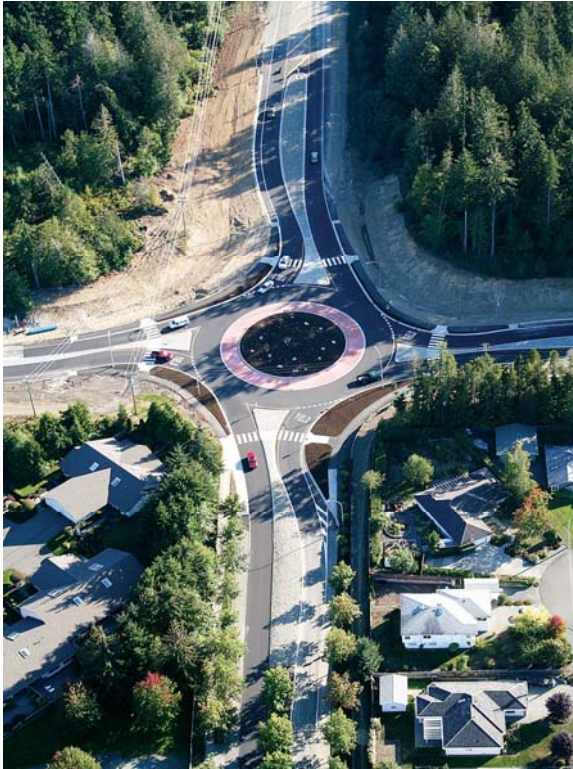
Aerial view of Roundabout looking south. The Roundabout has a 45 m inscribed circle diameter. (Photo courtesy Oceanside Star)
