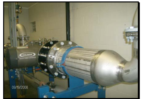
River Well UV Reactor Installation
