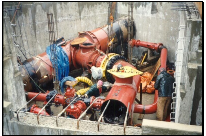
1200x1200x750mm dia tee and 750 mm dia.. butterfly valve c/w with 200 mm by-pass piping.
