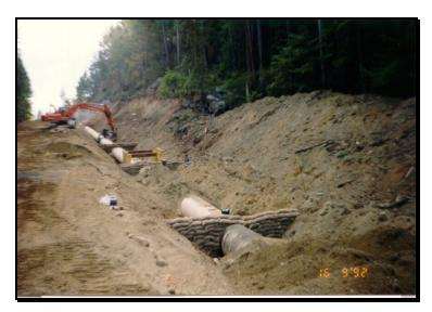
To prevent rapid migration of subsurface trench water and resulting erosion, concrete bag trench dams were constructed on grades over 10 percent.
