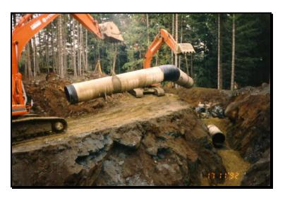
Excavators work together to lower in one of the 45 degree bends. This section was at the highest point on the supply main alignment and consequently the trench was excavated deeper than normal to optimize pipe capacity for gravity flow.
