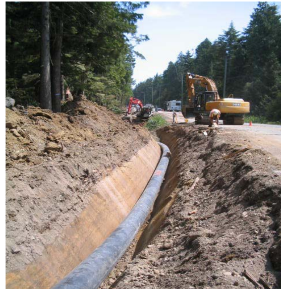
400 mm diameter HDPE pipe being installed in the road shoulder of the Pacific Rim Highway
