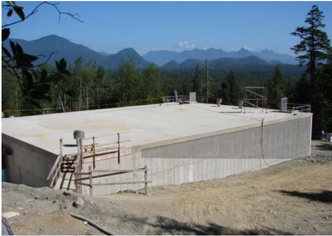
Completed reservoir looking northeast across Clayoquot Sound
